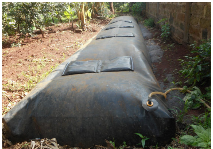
A biodigester—a prefabricated container that converts farm waste into organic fertilizer and clean fuel—in rural Kenya. Photo credit: Root Capital.
